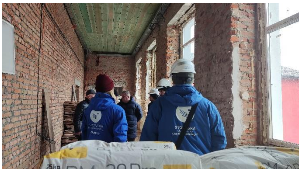
Zahal'tsi school renovation
